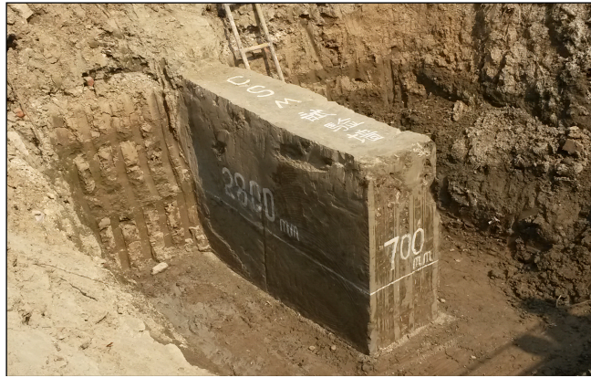
Figure 10. A trial CSM wall panel
