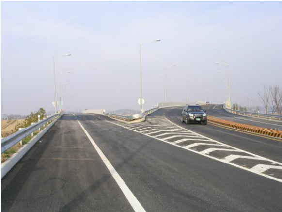
Figure 4. Remedial works at abutment
