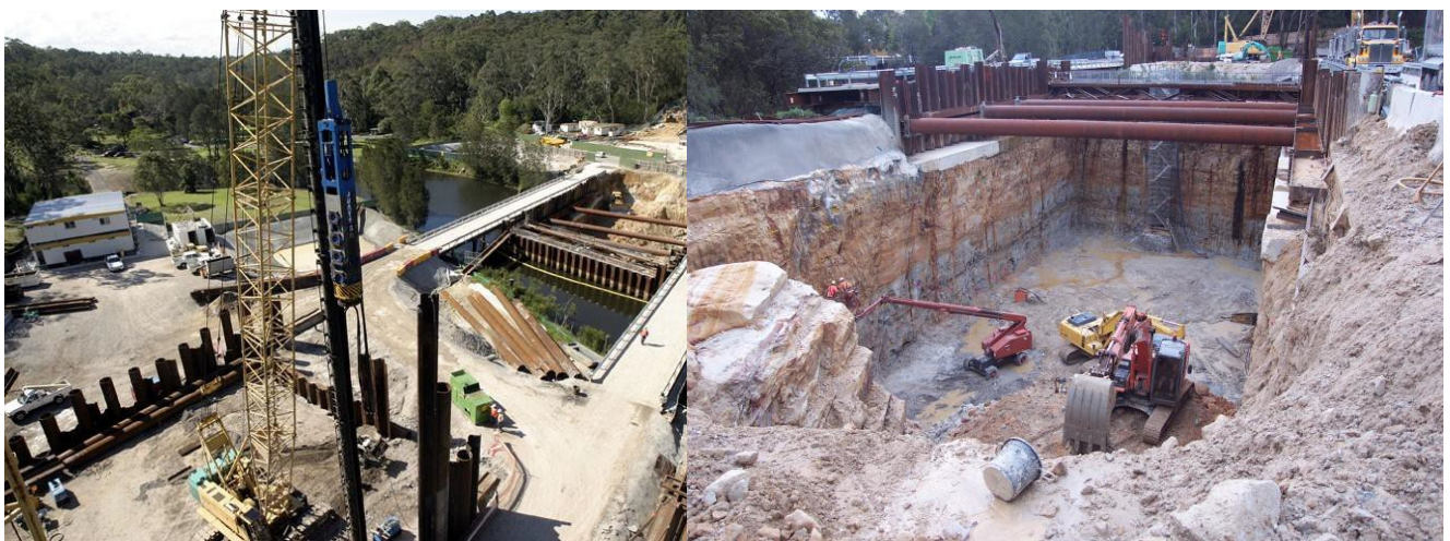
Figure 6. High-pressure grouting permitted safe excavation at Lane Cove River crossing
